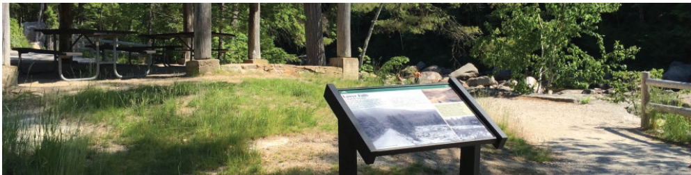
Installation of Interpretive Signage
